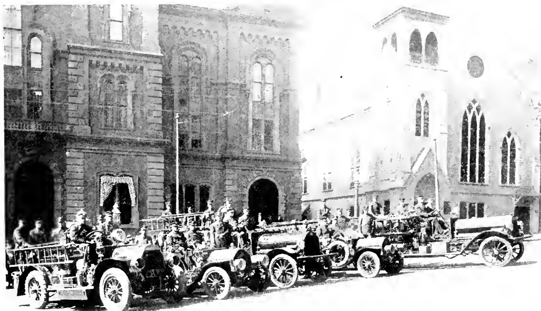
The Haverhill Fire Department is now completely motorized and is as up-to-date and efficient as any in the country. This picture shows only a part of the apparatus. (City Hall and First Methodist Episcopal Church in the background.)
